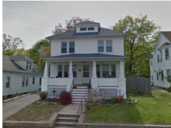
This property at 60 Lockhart Avenue was rehabilitated using HOME funds from the U.S. Department of Housing and Urban Development (HUD). © Google Maps.
