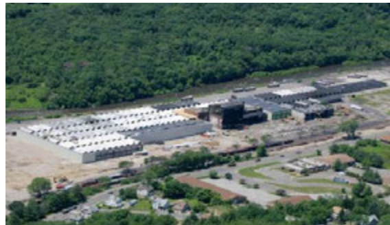
The Waterbury Industrial Commons in Waterville is one of the city's largest industrial areas. © WDC
