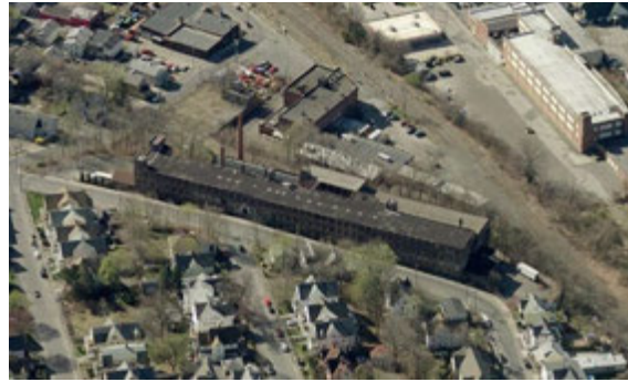
The Lux Clock Factory on Johnson Street is an industrially-zoned brownfield in a residential neighborhood. Expanding permitted commercial and residential uses could create greater flexibility in redeveloping the site. © Bing Maps
