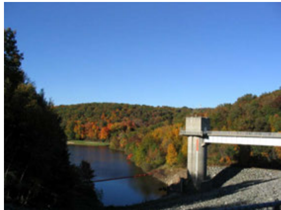
The Hop Brook Greenway would link Waterbury's open space system to the surrounding towns of Middlebury, Naugatuck, Oxford, and Southbury. © US Army Corps of Engineers
