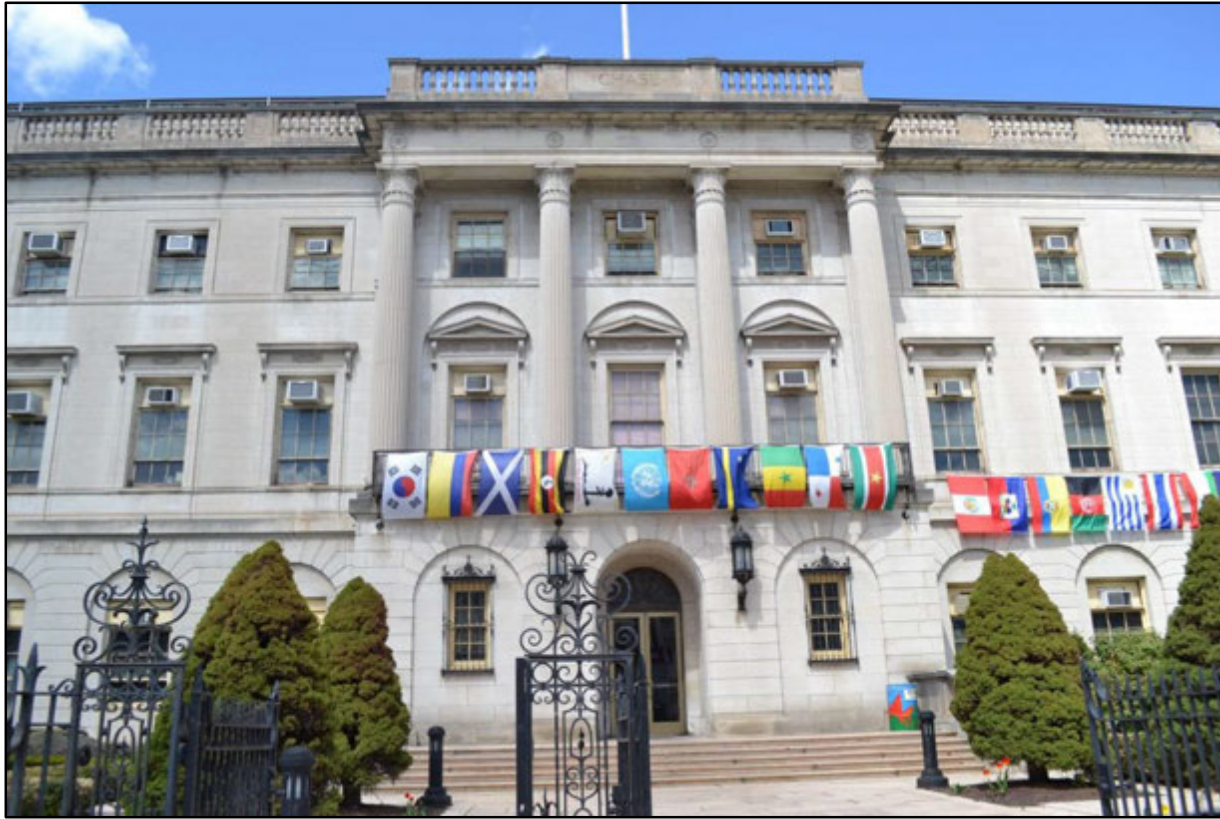
Chase Municipal Building
