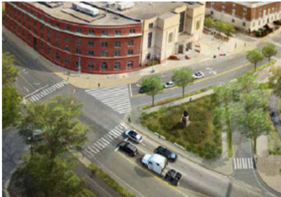
Pedestrian and bicycle accessibility to the train station will be greatly improved when the W.A.T.E.R. Project is completed © RBA Group
