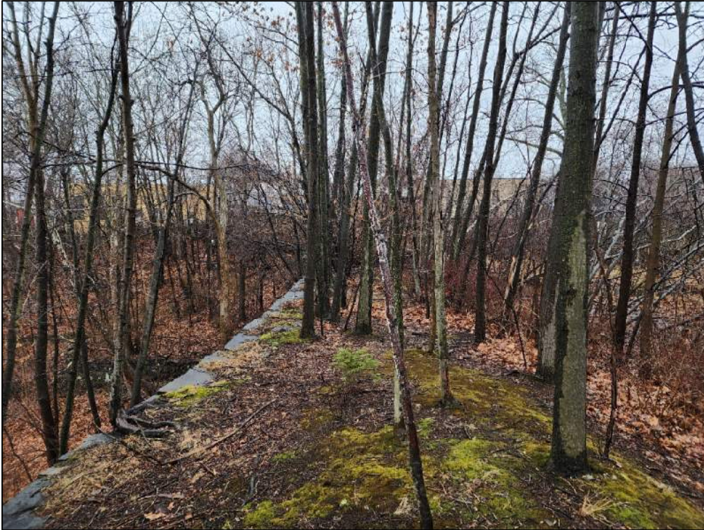
Photo 5 – Overview of dam crest from south end
