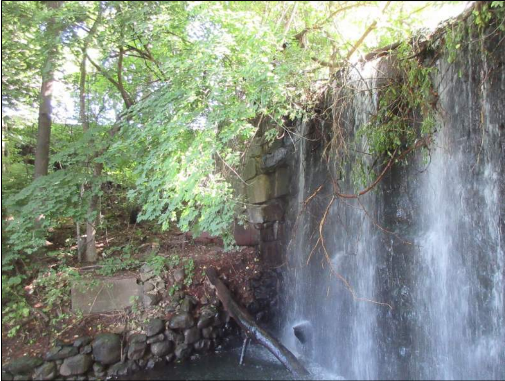
Photo 3 – Overview of downstream face of spillway and north side of dam
